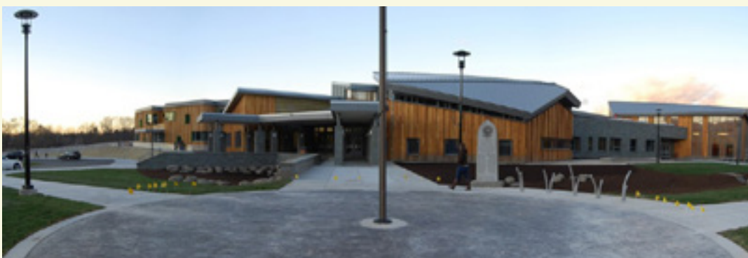
New Mac Arthur Elementary School, 1123 Vestal Avenue
